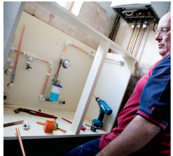
Above: Push-fit connectors can be used with copper pipe; but they tend to be larger and less attractive than traditional versions, so are best kept out of sight
